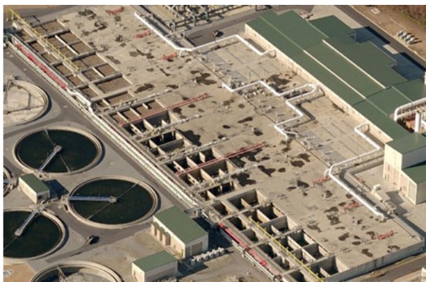
F. Wayne Hill WRC Biological Treatment Basins
